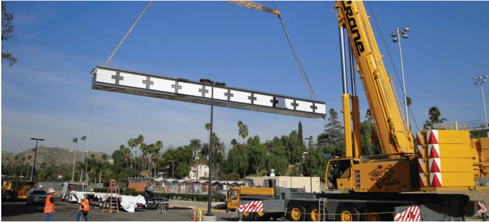
Installation of Natare Movable Bulkhead System at Riverside Aquatics Center, California.
