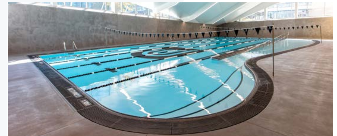
Deck level with S/S hand hold and integral deck drain
